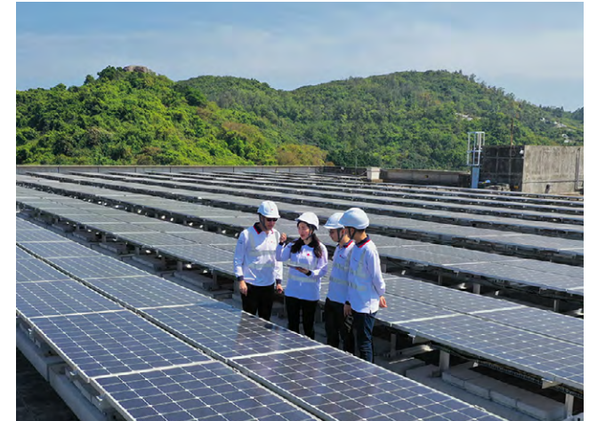
200 kW capacity solar installation at Gammon Technology Park in Tseung Kwan O.
