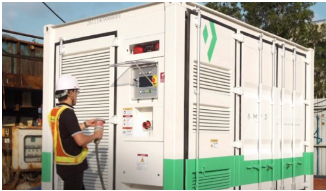
Using a battery energy storage system – the Enertainer.
