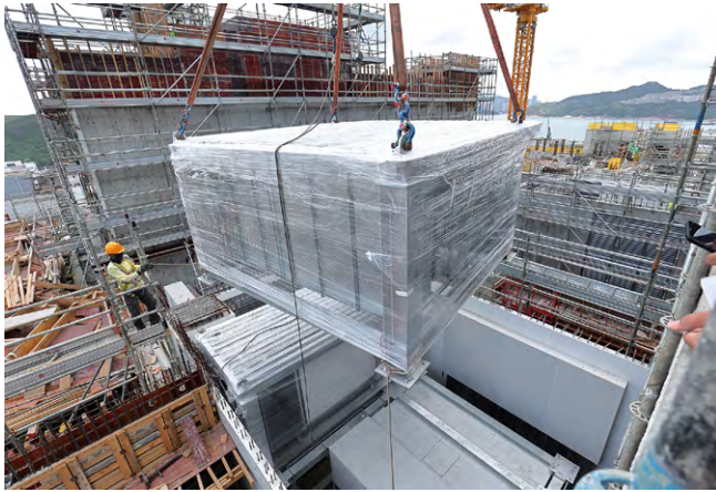
An MiMEP plant room is lifted into position.
